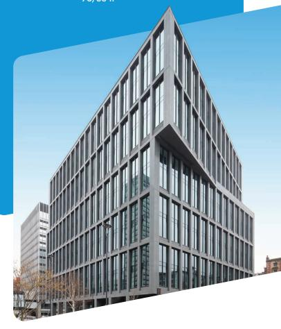
neutrality in transmission and exterior reflection distinguishes it as the most neutral coating within the COOL-LITE® XTREME range. The COOL-LITE® XTREME 70/33 is a triple silver coated glass with high solar control selectivity that does not compromise on aesthetics or cause glass distortion.
