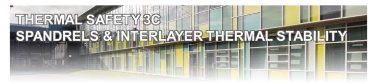
Spandrels and shadow boxes are typically used to conceal regions of the building containing utilities (pipes/cables) or structural elements, whilst still maintaining the appearance of a full glass façade. Spandrel units will typically have an opaque pane, and insulation in contact with the rear of the glazing unit, either adhered to the glass or secured in metal trays.
