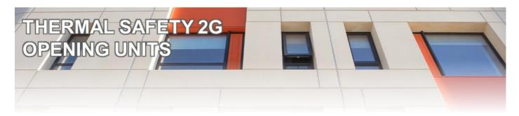
The thermal safety of units that open, whether pivoting or sliding, must be considered separately to vertical units, and will typically be based on worst case conditions, depending on allowable movement.
